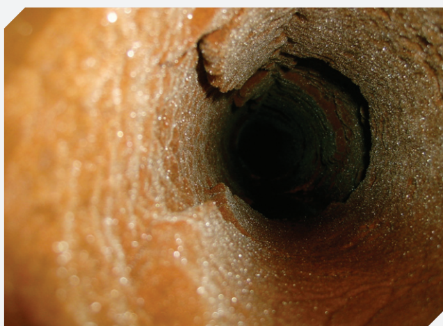
BEFORE PIG DESCALING
