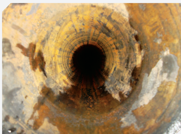
AFTER PIG DESCALING
